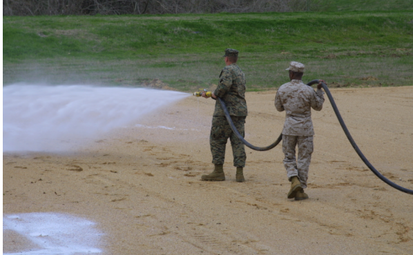
Photo 3. Spraying helipad using hand-held hose
