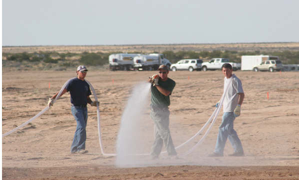
Photo 7. Spraying emulsion with hand-held hose
