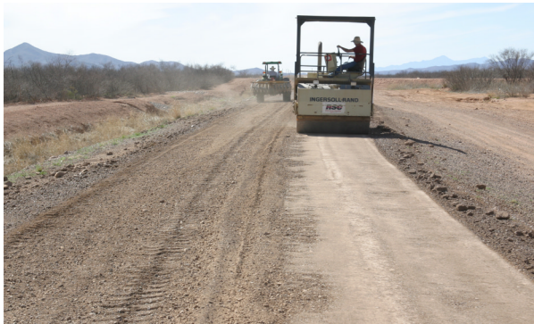
Photo 11. Compacting road surface after tilling (step g )
