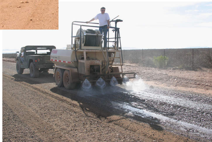
Photo 14. Applying synthetic fluid to road surface using distribution bar on rear of HydroSeeder
