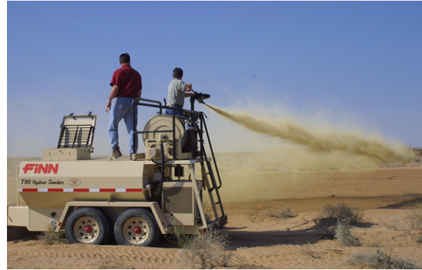
Photo 6. Distributing emulsion onto heliport using tower gun
