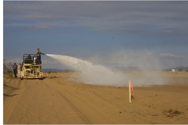
Photo 2. Spraying helipad using tower gun (step d )
