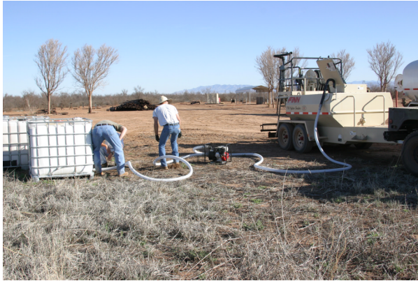
Photo 1. Filling HydroSeeder with product (step b )
