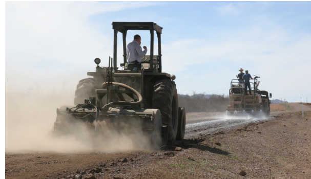
Photo 10. Applying product to road surface and distributing with rotary mixer (steps e,f )
